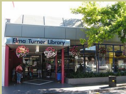
Elma Turner Library— Now using GO-GO PC control system
